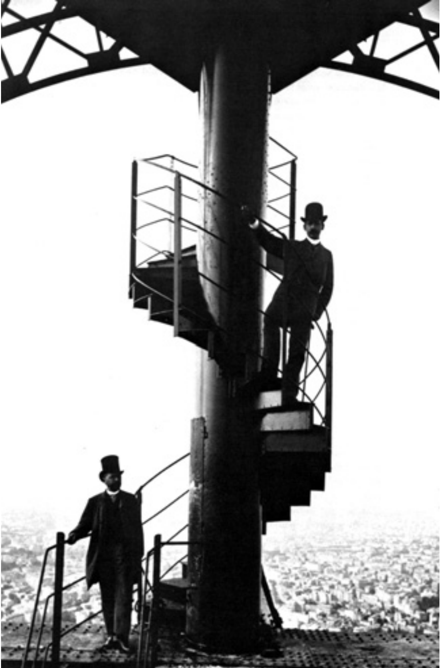
On completion of his tower, Eiffel poses with his son-in-law, Adolphe Salles, on spiral staircase. (Collection Viollet)
